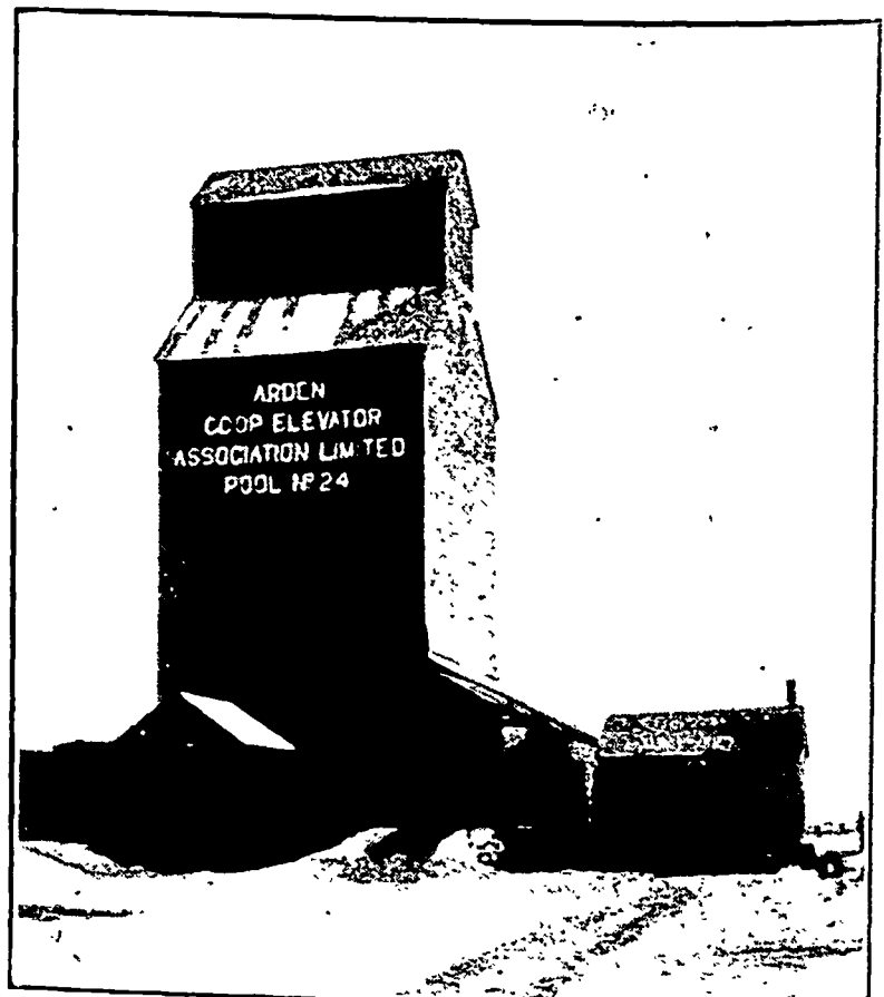
A TYPICAL POOL ELEVATOR.
